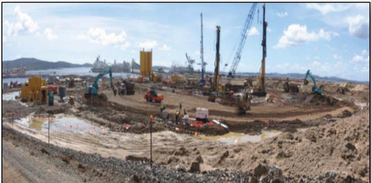
**Figure 2:** Site Construction at Fisherman's Landing (March 2010) showing Earthworks and Tank Piling Deep Soil Mixing
