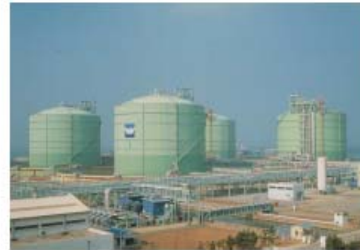
LNG regasification terminal in Pyeong Taek (10 x 100,000 m 3 )
